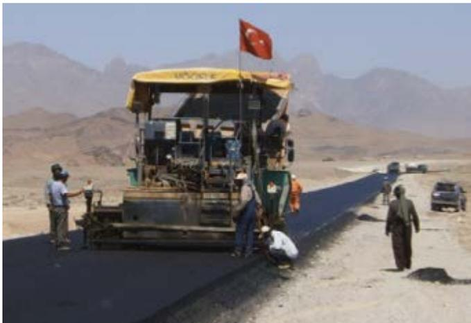
**Figure 7: Hot-mixed asphalt pavement plant on Keshim to Faizabad Road, Badakshan Province, Afghanistan**
